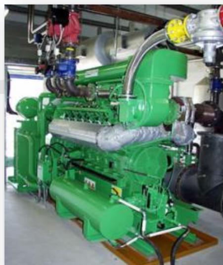
Picture 10 - Internal heat and power generation for grid independence
